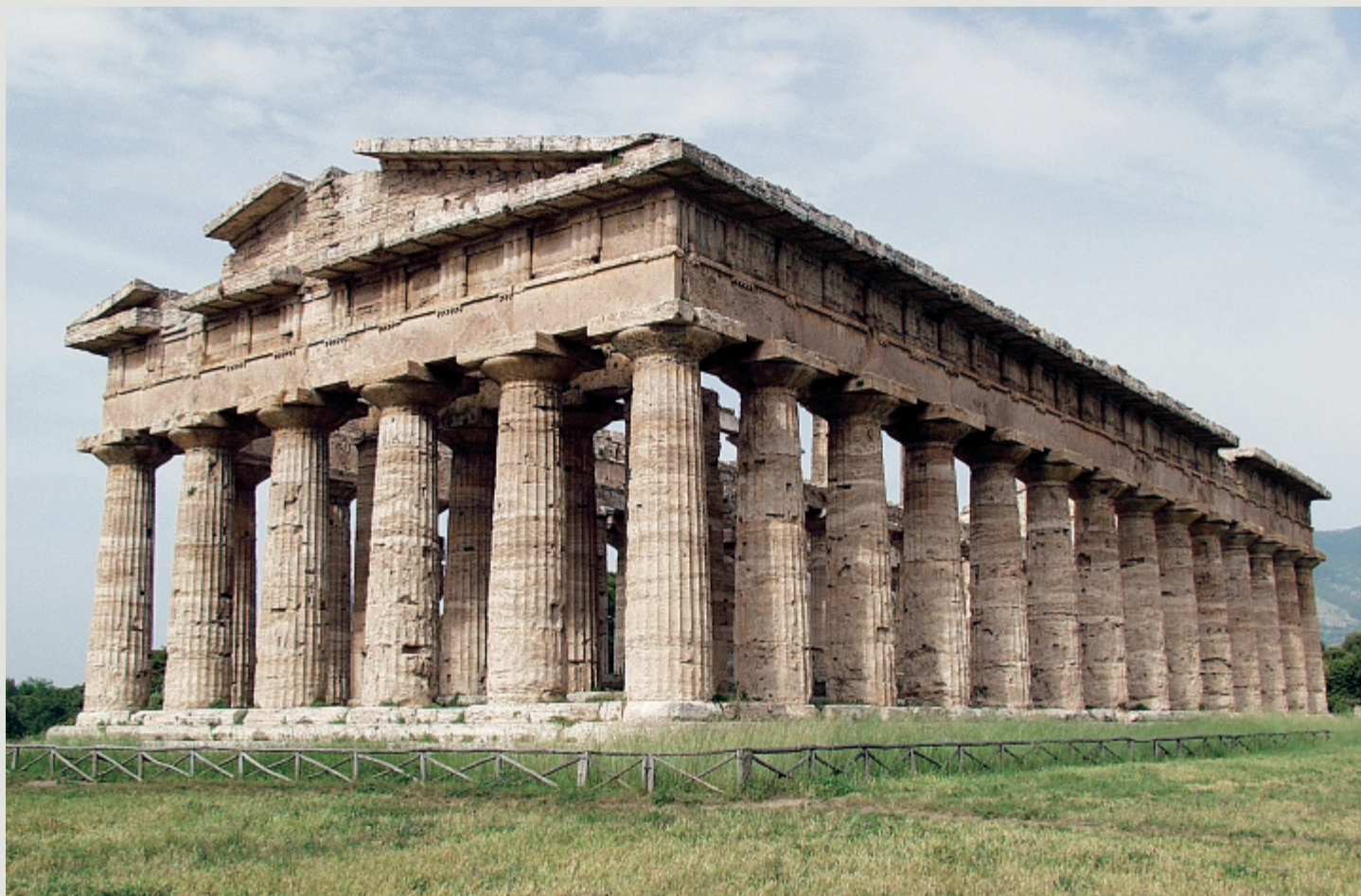
Greek Doric peripteral temple (Temple of Hera or Apollo, Paestum, Italy, ca. 460 BCE)
