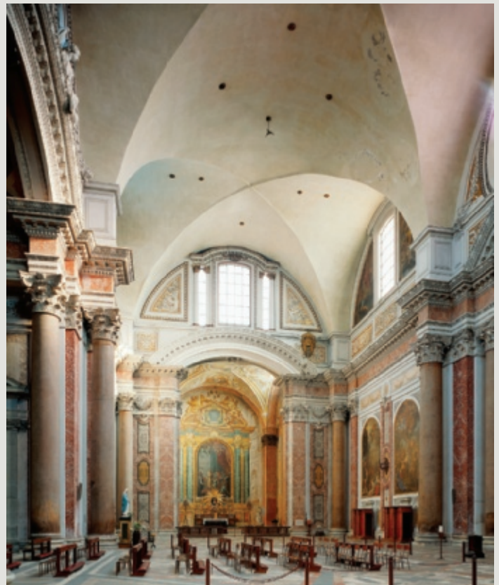
Roman hall with groin vaults (Baths of Diocletian, now Santa Maria degli Angeli, Rome, Italy, ca. 298–306)
