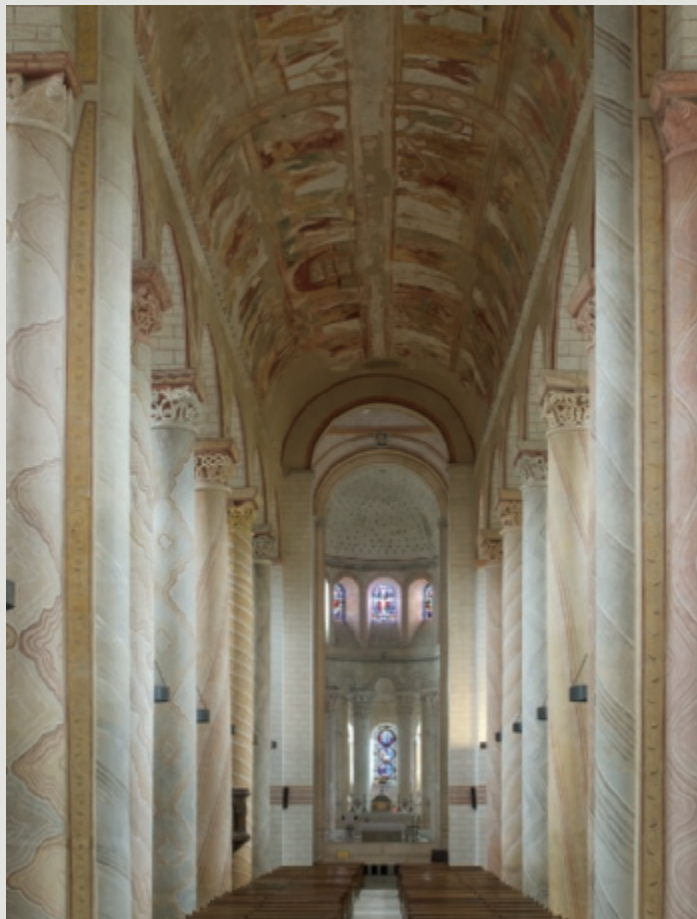
Medieval barrel-vaulted church (Saint-Savin, Saint-Savin-sur-Gartempe, France, ca. 1100)
